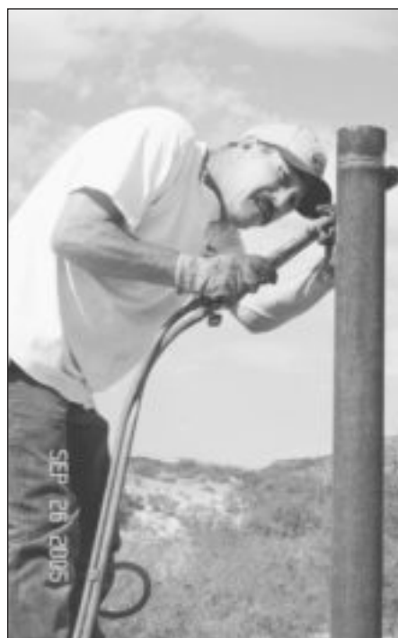
YAPD SERGEANT Cecil Bruno helps build the new bus stop for Middle Verde children at the intersection of Reservation Loop Road and Hamaley Street.
