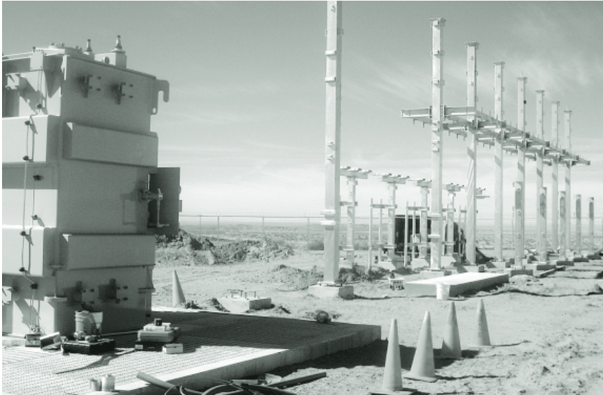
Substation equipment being installed at Shiprock, New Mexico
