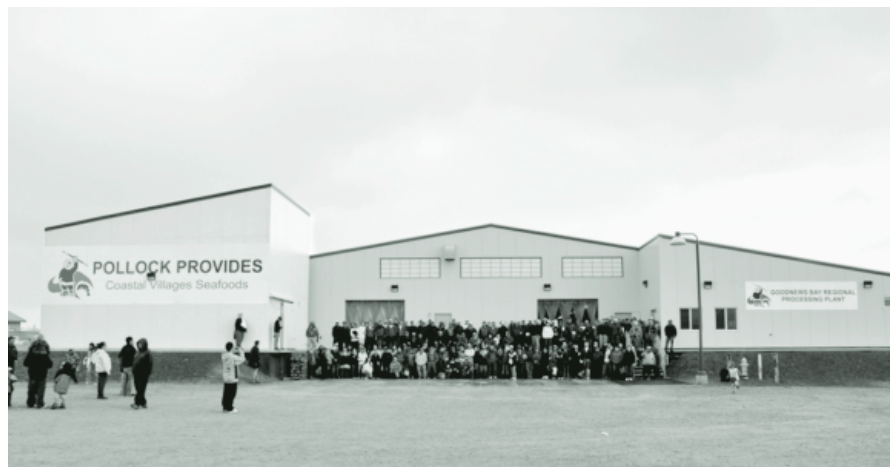
Grand opening of CVRF Processing Plant
