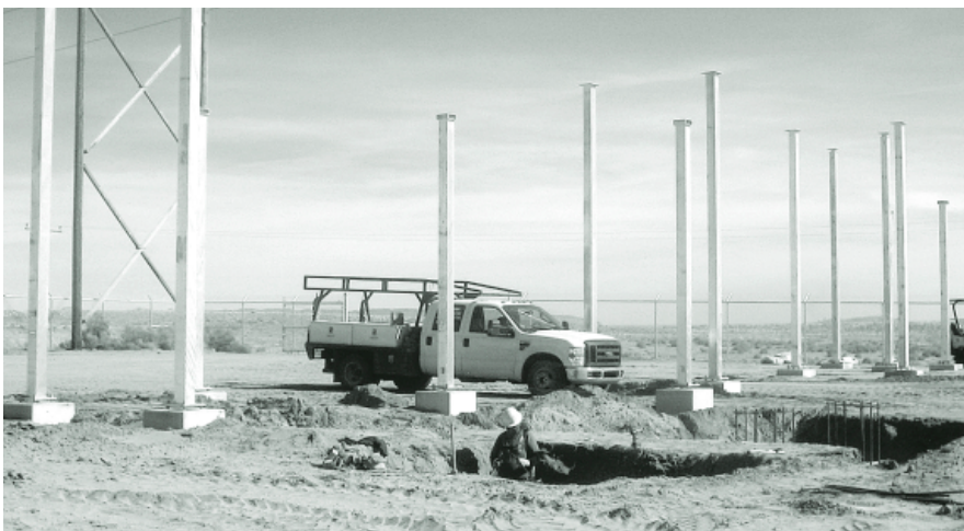
Transmission equipment being installed to tie into grid
